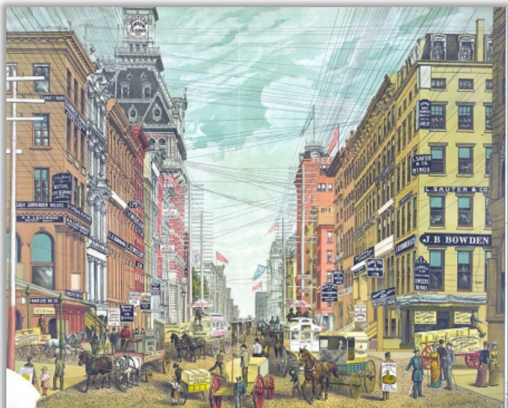
Lower Manhattan criss-crossed by wires As this 1880s postcard reveals, New York streets in the late 19th century held messes of wires—telephone and telegraph wires like these as well as power lines.
